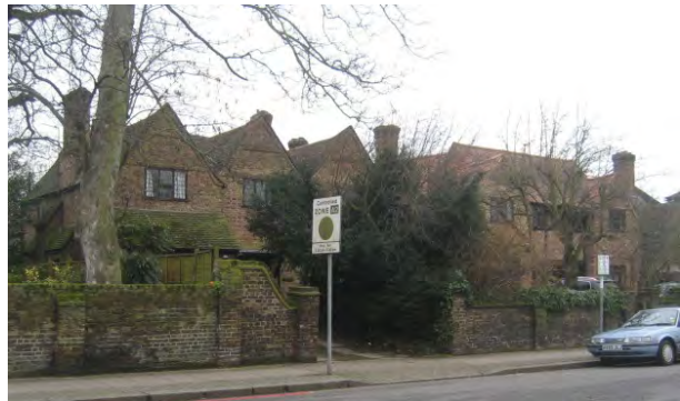
Figure 21 : Brown brick, gabled frontages and leaded light windows are further features of the Old English style
