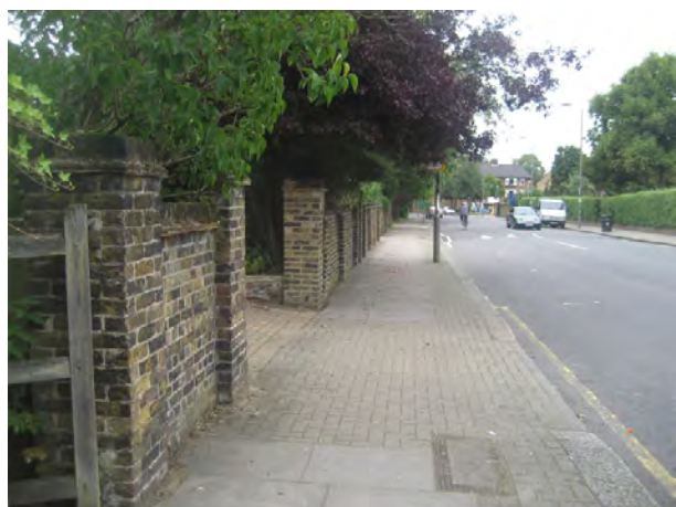
Figure 22 : The continuous boundary wall which is contemporary with the houses
