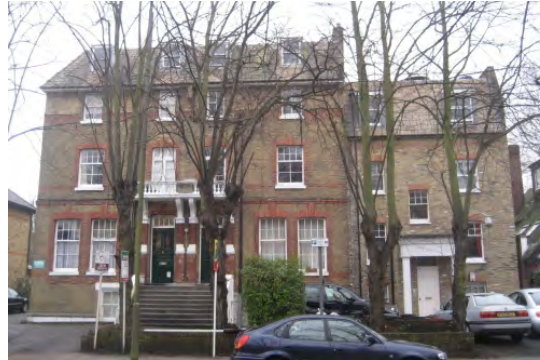
Figure 35 Pair of late Victorian town houses (extended to the right)
