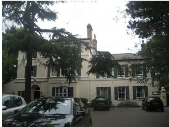
Figure 44 : The Pines Nursing Home (sub-area a)
