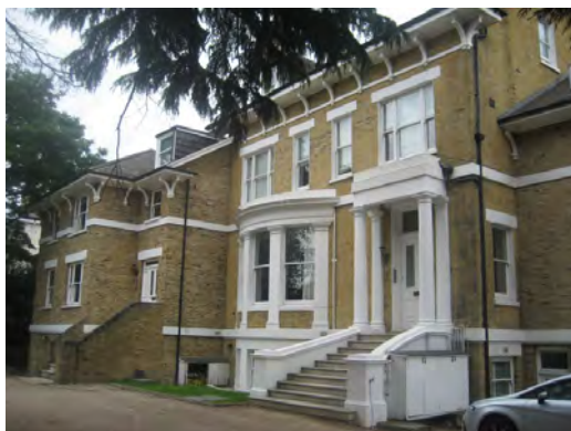
Figure 19 : Langton Court (extended on the left) seen from West Hill. The cottage style houses were built in its garden
