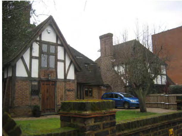
Figure 20 : The Old English style used vernacular details such as mock timber framing, tall chimneys and catslide roofs
