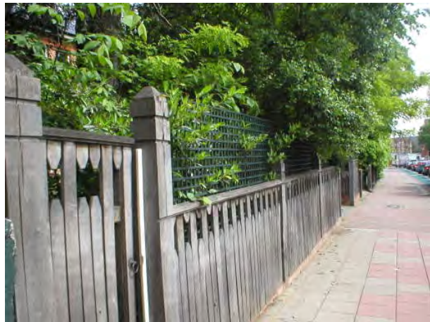
Figure 52 : Distinctive fence design at 88 West Hill
