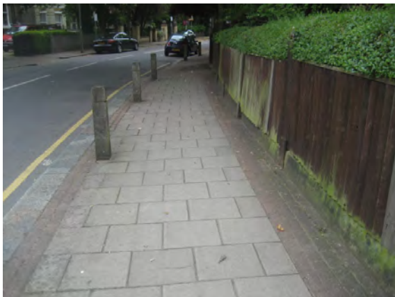
Figure 39 : Traditional fence outside Oakhill Court and traditional style slab paving
