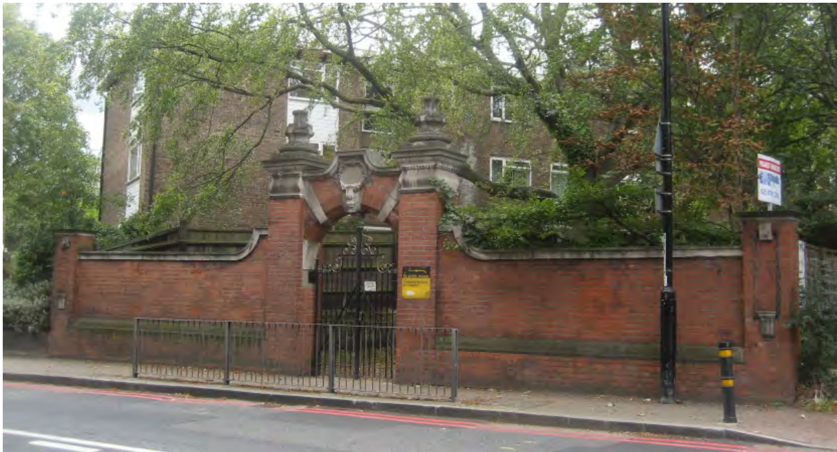
Figure 31 : Decorative gate and wall
