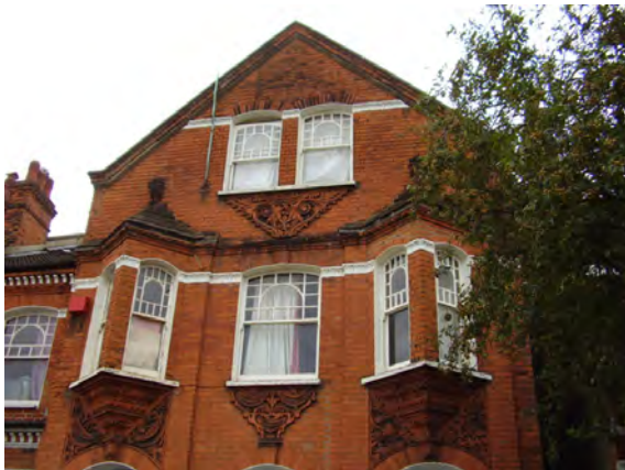
Figure 59 : Sash windows with distinctive glazing pattern in upper sashes
