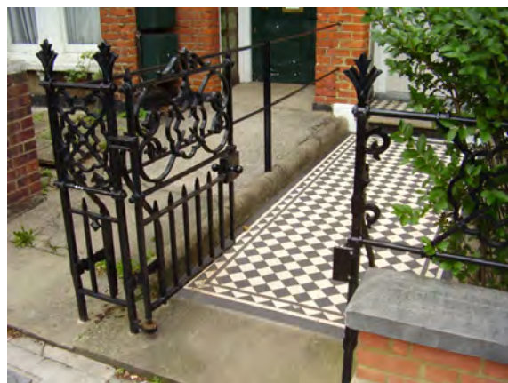
Figure 62 : Replica gate and original tiled path
