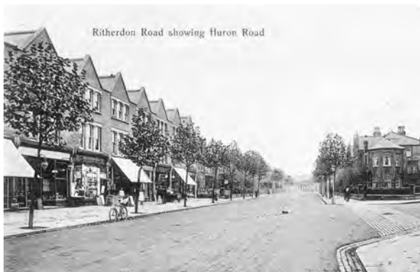
Figure 45 : Historic photograph of the shops at nos. 2-24 Ritherdon Road
