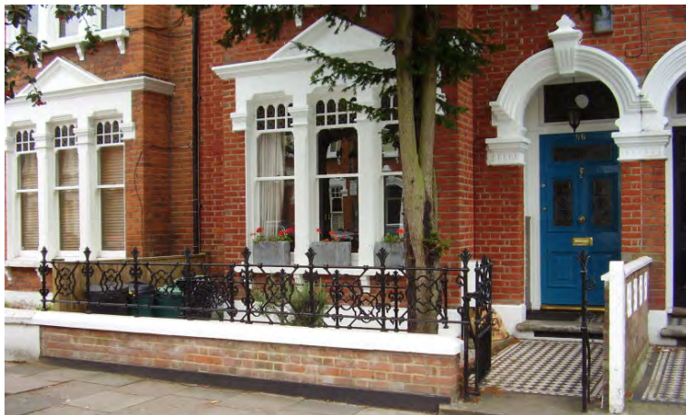
Figure 40 : Reproduction railings, original sash windows, front door and tessellated path in Louisville Road
