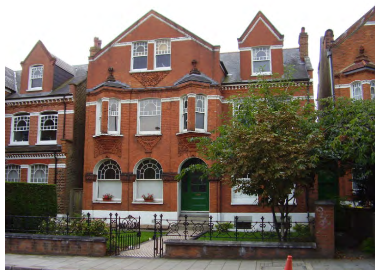
Figure 15 : A beautifully restored house on Bedford Hill
