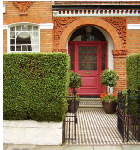
Figure 29 : Original front door, tile path, carved brick detail and replica railings
