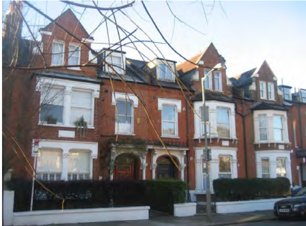
Figure 44 : Manville Road - where 'Group B' (right) meets 'Group C' (left)
