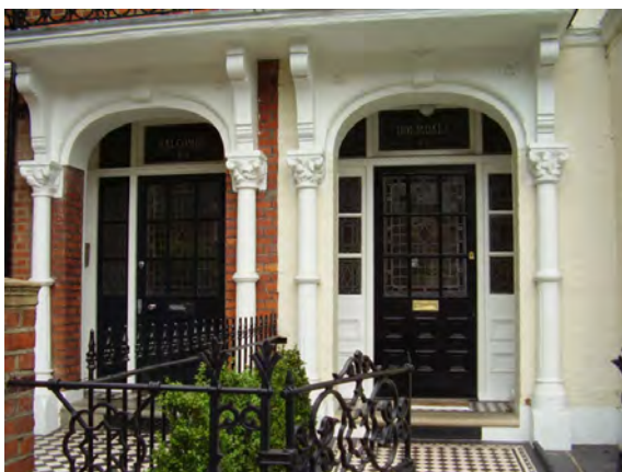
Figure 61 : Pair of original panelled doors with columned porches
