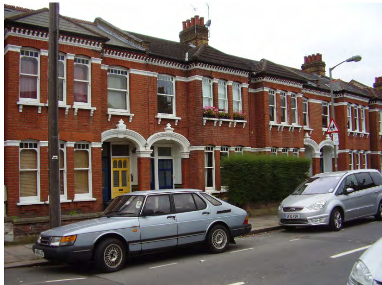
Figure 38 : 'Group E' purpose built flats - note the pairs of doors in shared porches
