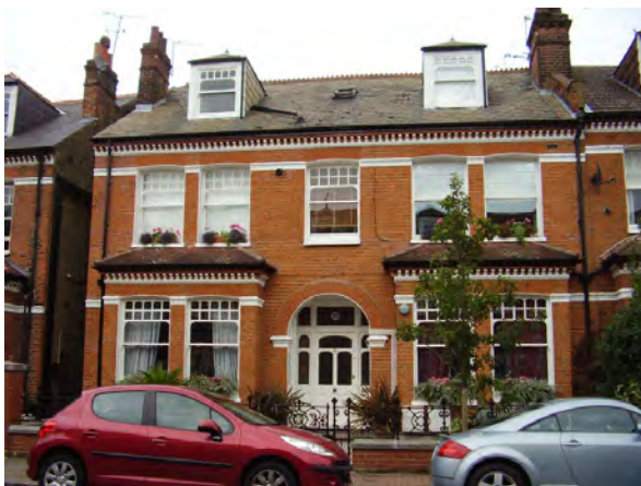
Figure 43 : 'Group A'. Double fronted house, note the door with matching sidelights and fanlight
