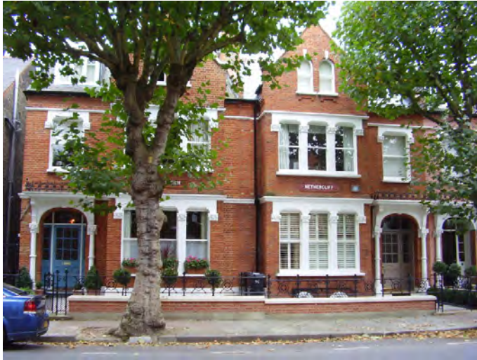
Figure 52 : 'Group A' houses with round headed gable windows and columned porches. Note the house names above the ground floor windows
