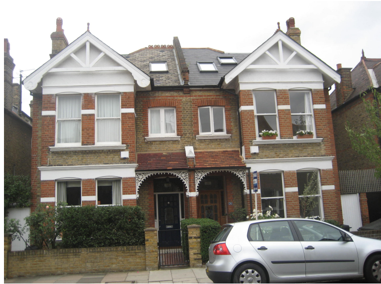
Figure 17 Pair of stock brick houses. Note the timber details in the gables and the decorative cast iron spandrels to the porches
