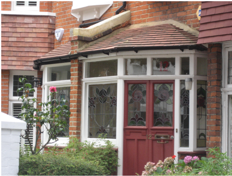
Figure 14 Close up of an original porch
