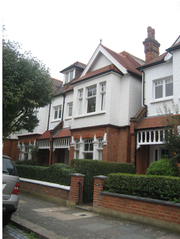
Figure 16 Group of red brick houses with rough cast to the first floors
