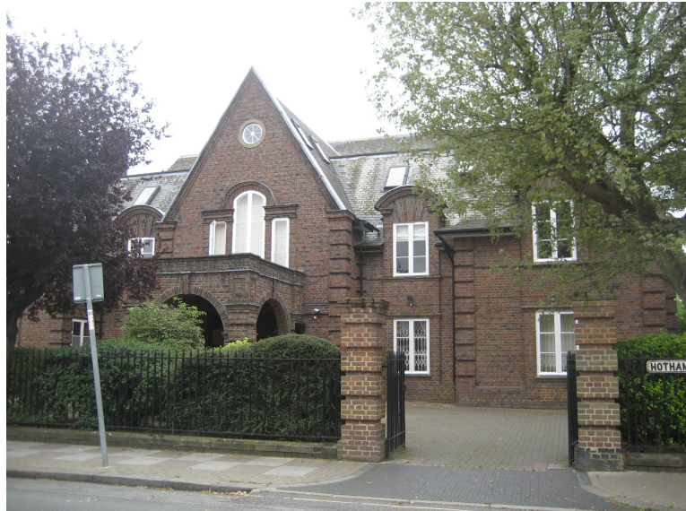
Figure 20 St Mary's Hall
