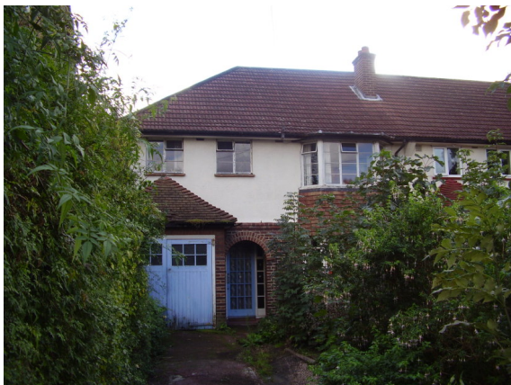
Figure 12 : No. 94. Built in the 1930s, this house has retained its original Crittall windows, front door and garage door
