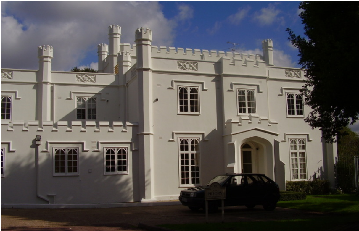
Figure 3 : The Priory (a Grade II listed building)
