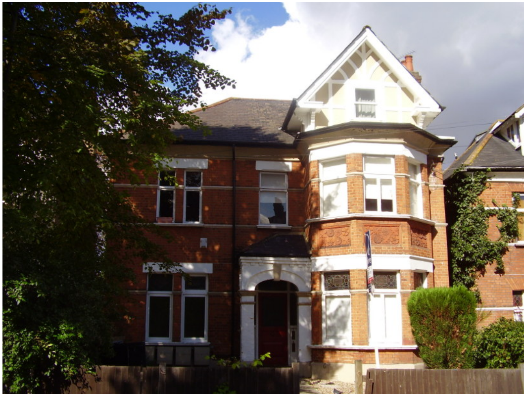
Figure 9 : The predominant house type on the northern side. A red brick detached villa with an asymmetrical full height bay with timbered gable and porch to the centre. Note also the tall windows and carved brick panels
