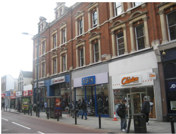
Figure 17 : Modern shopfronts with oversized fascias which fail to reflect the tall vertical proportions of the building above and in fact look squat and cramped
