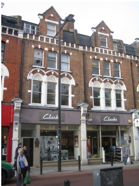
Figure 19 : New traditional style shopfronts have reintroduced the correct proportions and features for the building
