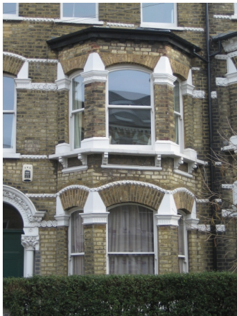
Figure 50 : Original plain sash windows
