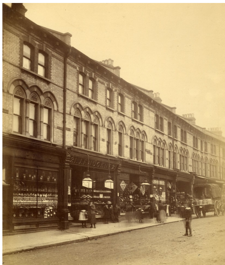
Figure 15 : Nos.19-27 St John's Road soon after they were built c.1890
