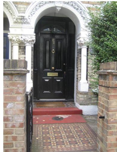
Figure 49 : Original front door and tile path with coal delivery hole
