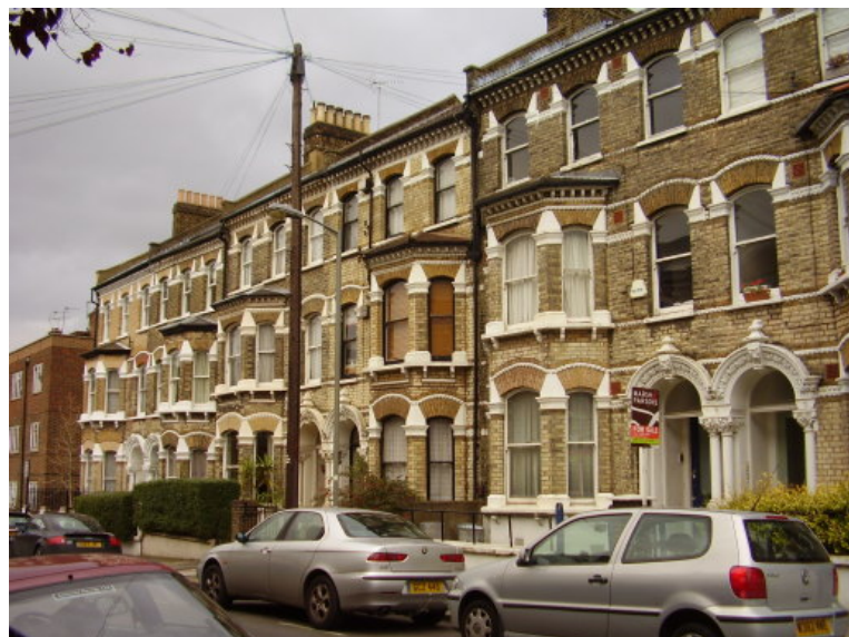
Figure 48 : Victorian stock brick terrace
