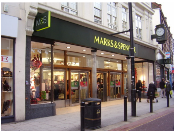
Figure 21 : The elegant interwar bronze shopfront to Marks & Spencer. The sign and canopy have been added but the slim glazing bars and steel columns are original
