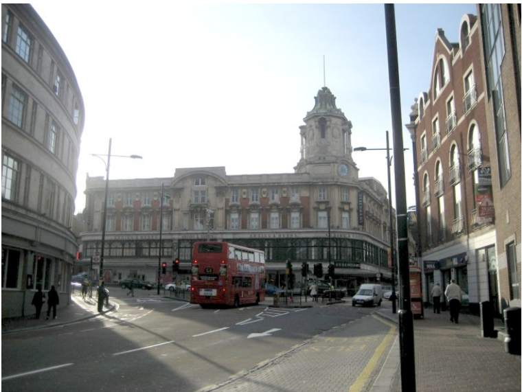
Figure 25 : The former Arding and Hobbs department store as seen today
