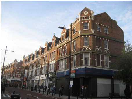
Figure 44 : Nos. 48-64 have gothic detailing. Some of this has been obscured by the concrete ring beams to the corner building
