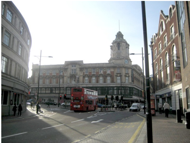
Figure 8 : Looking towards the historic space at the junction of Lavender Hill and St Johns Hill today marked by the tower of the former Arding & Hobbs department store
