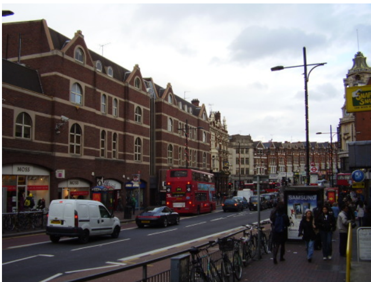
Figure 30 : Buildings containing the station booking office and shopping arcade. The scale of the building sits well with neighbouring buildings, but the design fails to reach the standard set by them
