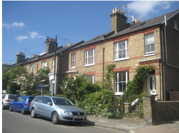
Figure 56 : Houses on the west side of Redgrave Road with red brick dressings and tripartite windows
