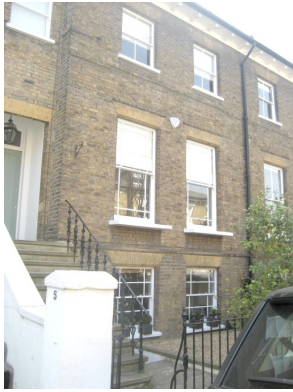
Figure 45 : Original sash windows with different glazing pattern on each floor
