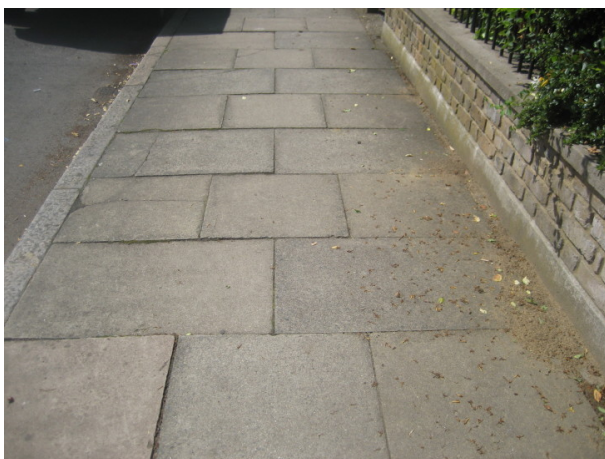
Figure 66 : Traditional style paving slabs in Redgrave Road
