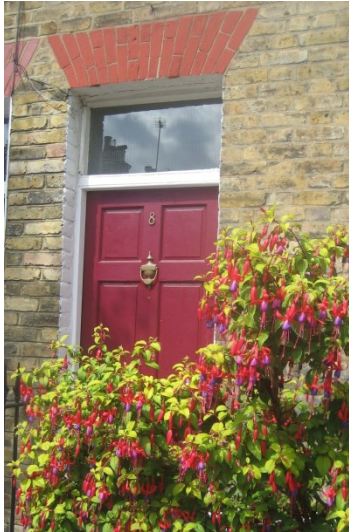
Figure 72 : Six panelled door on Lifford Street
