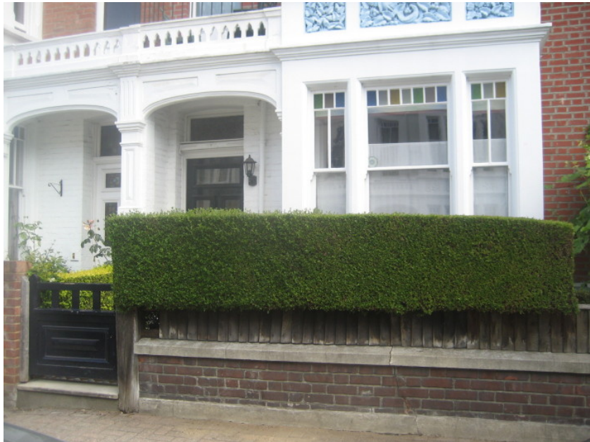
Figure 53 : An excellent original style boundary in Chelverton Road: red brick wall with coping stone topped with a short feather edged fence, neatly clipped privet hedge and wooden gate
