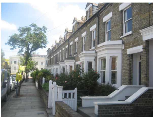
Figure 55 : 1-35 Redgrave Road (east side)
