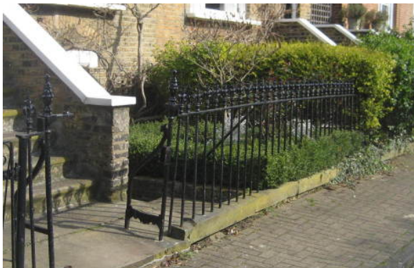
Figure 48 : Original railings with Fleur de Lys finials
