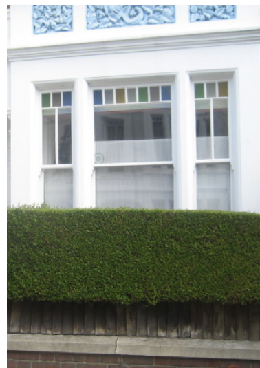
Figure 71 : Another window type in Chelverton Road
