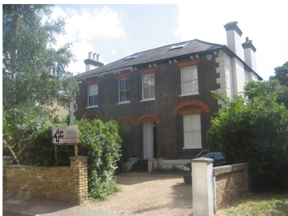
Figure 15 : Brown brick villa pairs with chimneys to the sides
