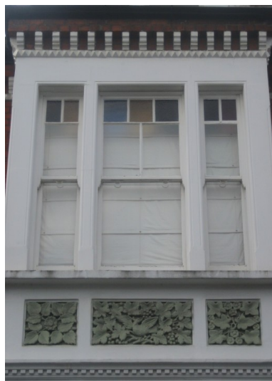
Figure 70 : Sash window from Chelverton Road
