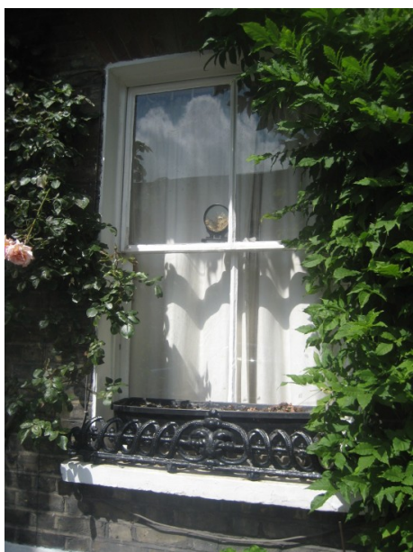
Figure 68 : Sash window with central glazing bar (note also the original cast iron window box guard)
