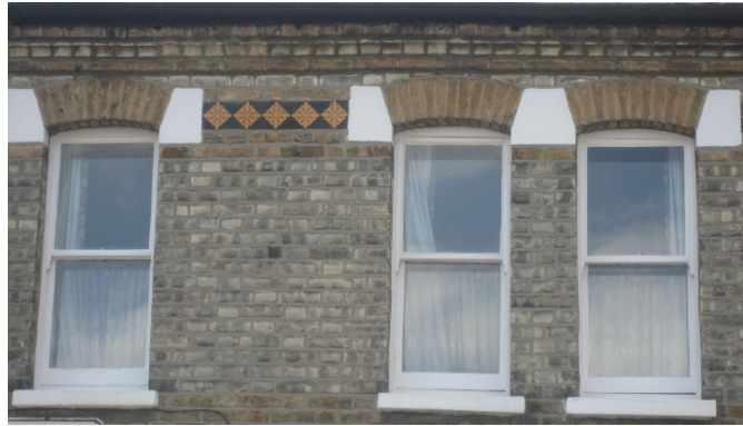
Figure 65 : Decorating tiling under the eaves
