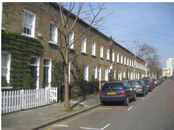
Figure 31 : The terrace on the west side of Lifford Street
