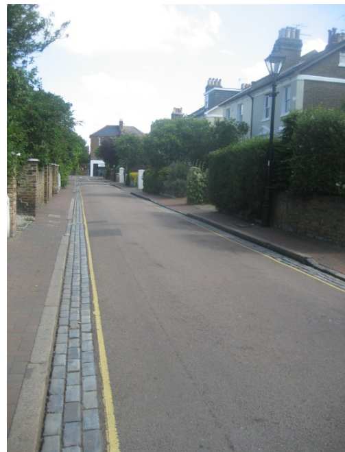
Figure 24 : View northwards showing the granite gutters and kerbs and well planted front gardens
