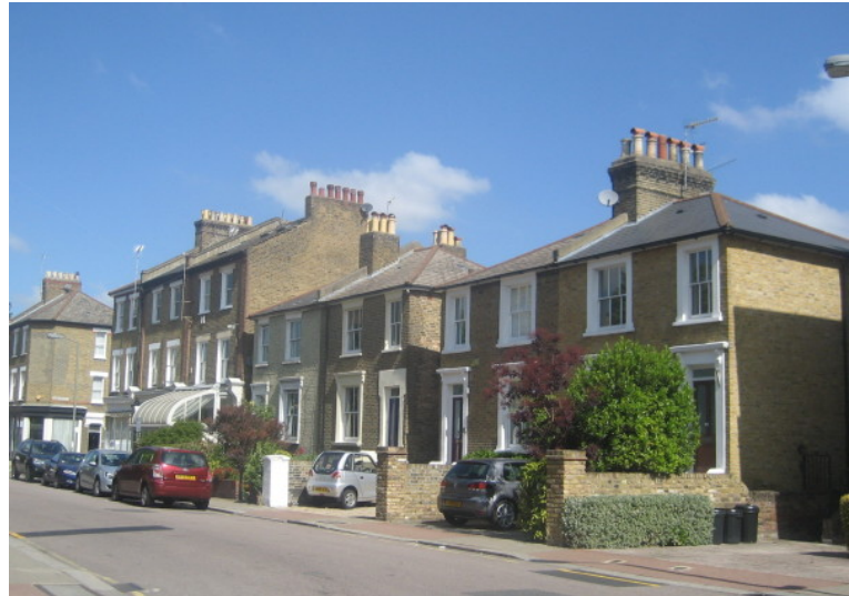
Figure 61 : 88-100 Felsham Road with the two villa pairs are in the foreground at no. 88-94
