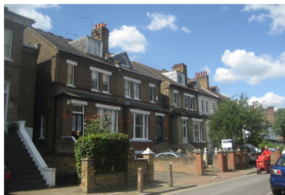
Figure 22 : 11-19 Clarendon Road today. Note some of the triangular dormers survive as do some pillar caps but the old boundary walls and hedges have been lost
