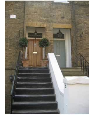
Figure 47 : Original front doors with two long flush beaded panels. (Paint is the correct finish)
