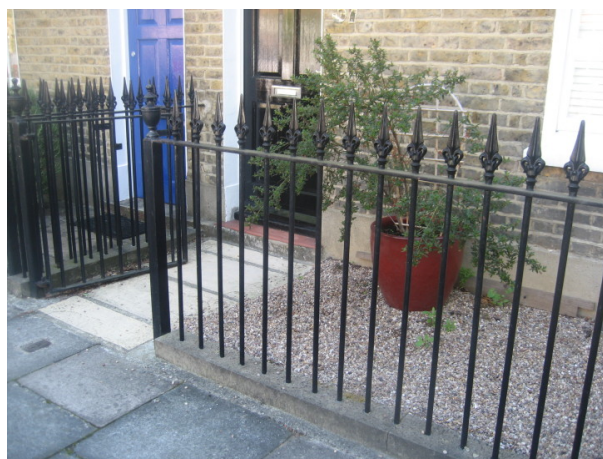
Figure 40 : Copies of period railings in Lifford Street
