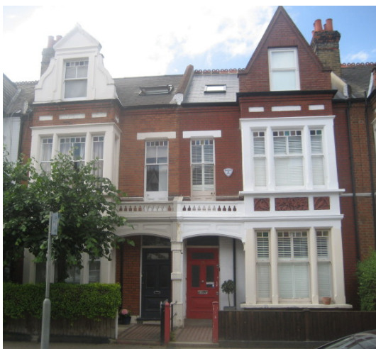
Figure 50 : A pair of houses in Chelverton Road. Note the different gable designs and the stone balustrade above the porch
