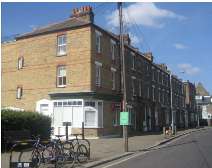
Figure 57 : 77-91 Lacy Road - all former shops now converted to residential accommodation
