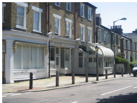
Figure 63 : The conservatory that breaks up the terrace frontage
