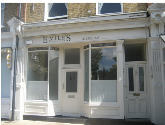
Figure 62 : This historic shopfront at no. 98 makes a good entrance for the restaurant but sadly the conservatory extension next to is rather incongruous
