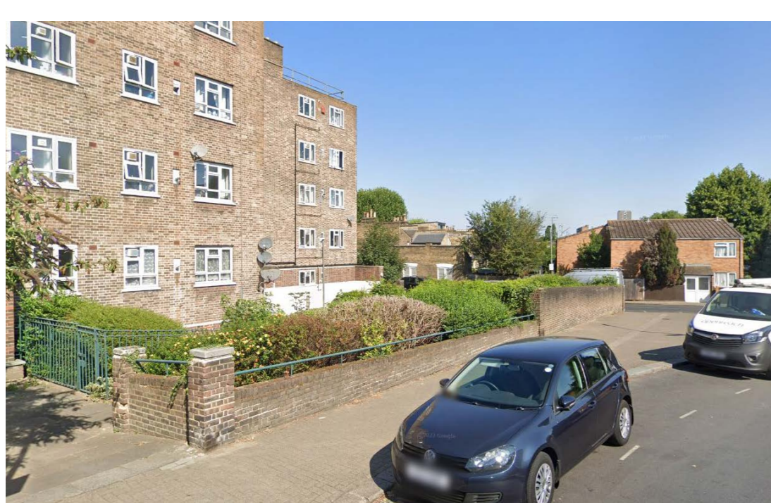
4 East view from Ashley Crescent
