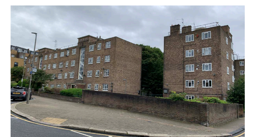
Photo 05. Retaining Wall Between Block B Site And Street
