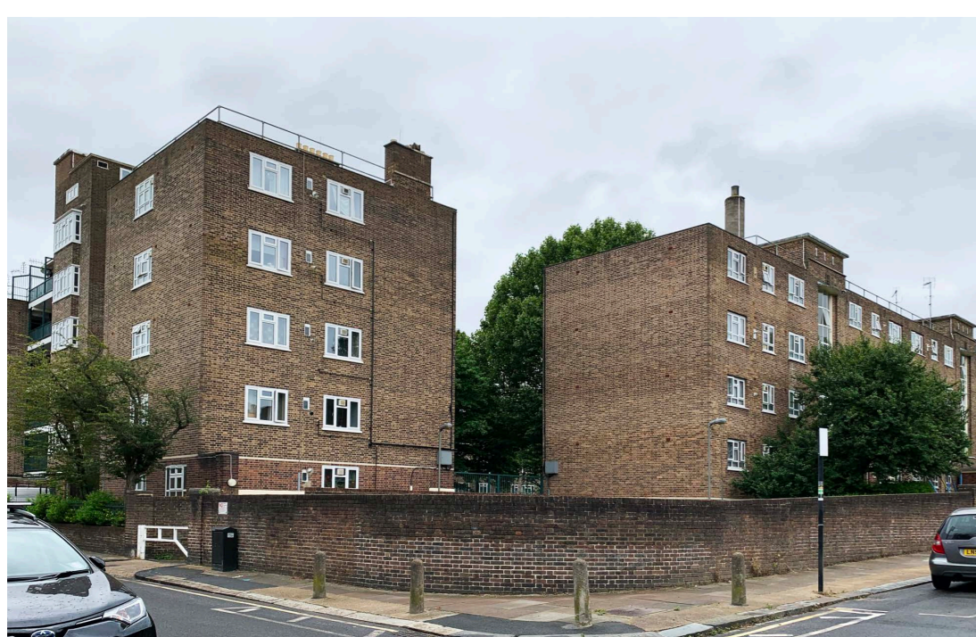
1 North-West view from Shirley Grove
