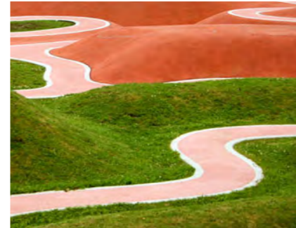
Resin bound paths & Lawn Type: Resin Bound Natural Aggregate 6mm & Reinforced turf
