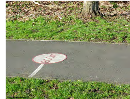
Trim Trail Element A Type: Thermoplastic line markings to denote distance on the footpath.
