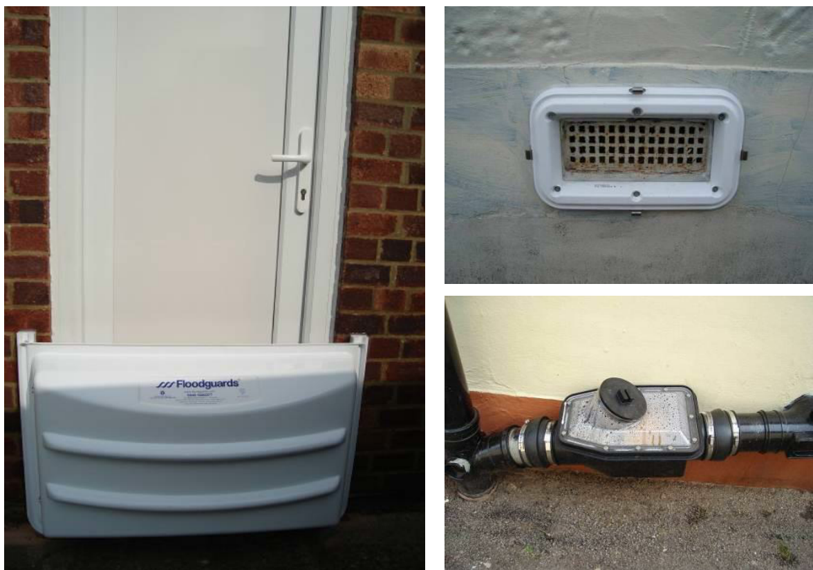
Figure D-2 Examples of flood barriers, air bricks and non-return valves
