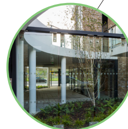
Well defined entrances to stairwells and communal areas
