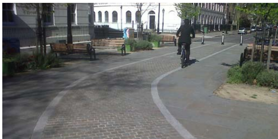
Bollards are highly visible while being sympathetic to the local streetscape
