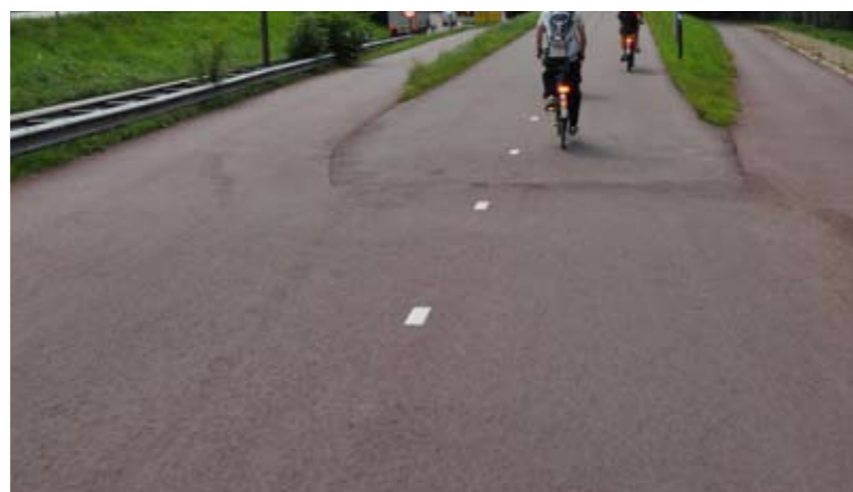
Surfacing needs to be immediately recognisable as a place for cycling. It should be smooth, with good grip and of high quality construction.
