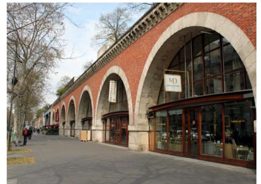
Development of railway arches enhances the streetscape
