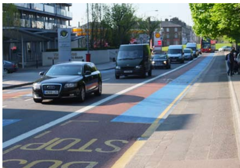
1 5 CS 8 (carriageway) and LCN 5 (footway)
