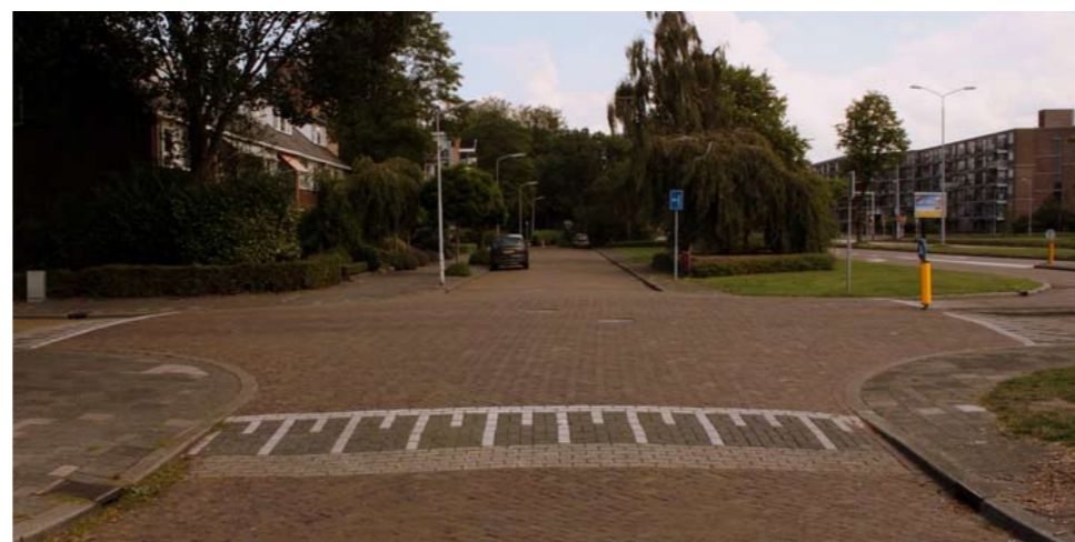
Traffic speeds at raised tables can be controlled via tight junction geometry
