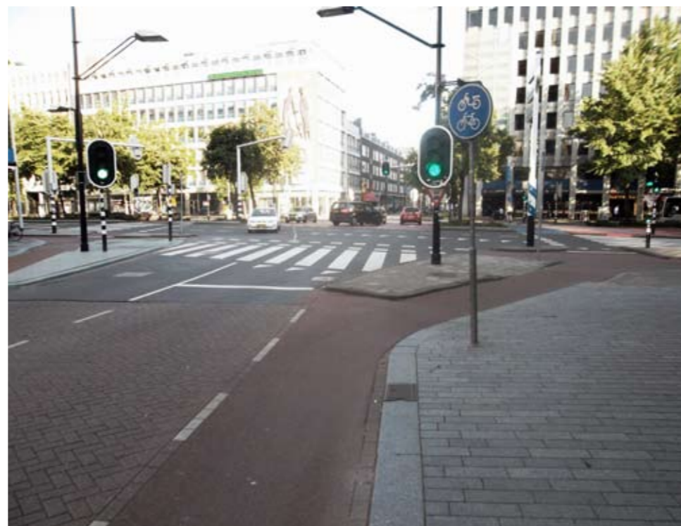
Refuge lanes at junction with main road; lanes must have sufficient capacity for expected levels of cycle traffic
