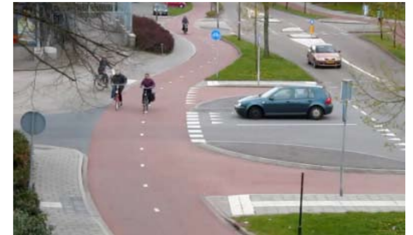
Cycle tracks continuous through side roads - turning traffic gives way
