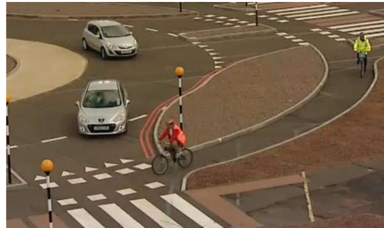
Cycle tracks segregated through roundabouts (undergoing trials)
