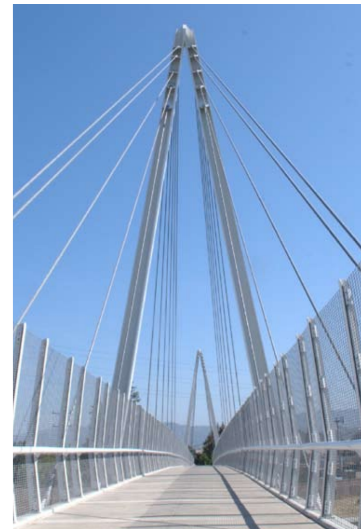
Pedestrian and cycle bridges overcome barriers of water and rail
