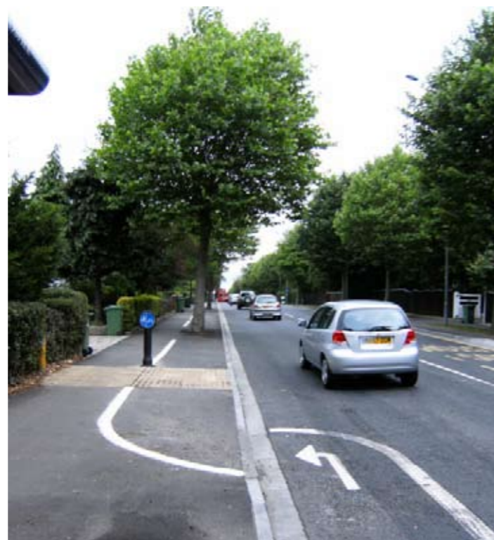
Abrupt, inconsistent lane treatments
