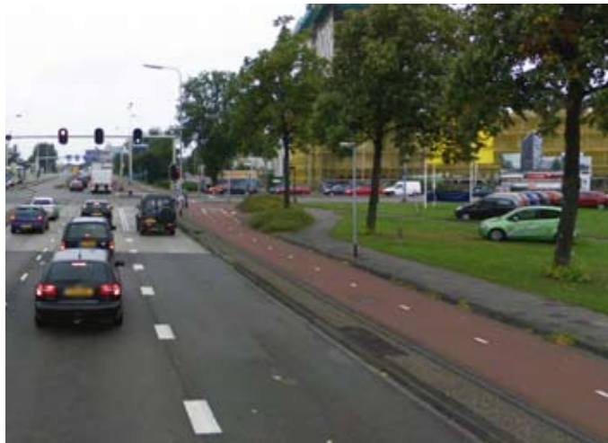
Kerb segregation provides high levels of subjective safety and is widely used in the Netherlands
