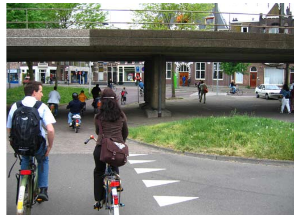
Cycle path continues under road bridge
