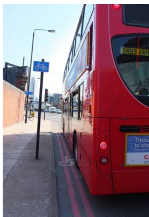
Unsafe on-carriageway provision
