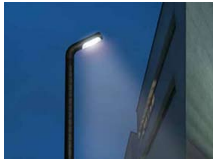
Light fittings should be high quality and attractive
