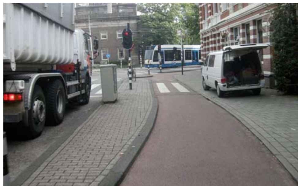
Kerb provides protection from HGVs at junctions
