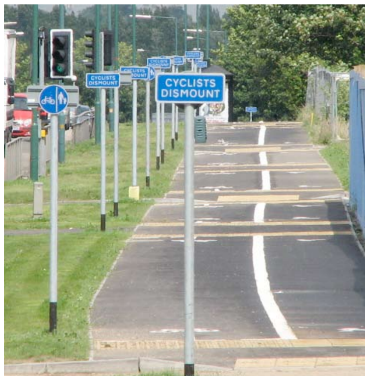
Lack of priority at side turnings
