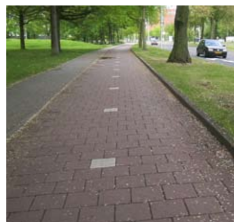
Surfacing needs to be immediately recognisable as a place for cycling. It should be smooth, with good grip and of high quality construction.
