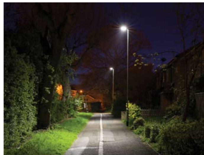
Lighting allows the tracks to be used 24 hours a day
