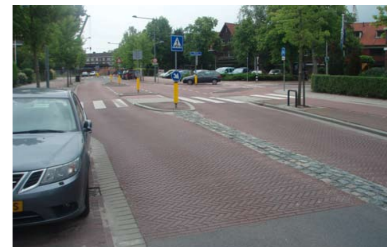
Pedestrian crossing with wide island accommodates bicycles
