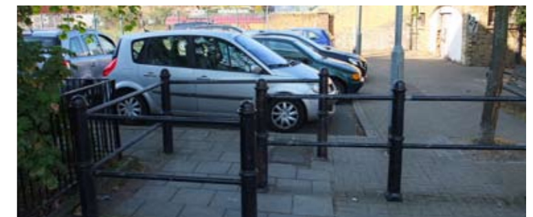
At-grade access restricted by barriers and car parking
