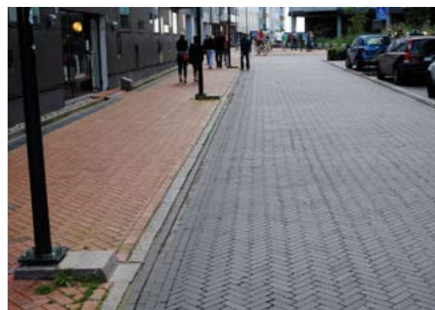
Surfacing needs to be immediately recognisable as a place for cycling. It should be smooth, with good grip and of high quality construction.
