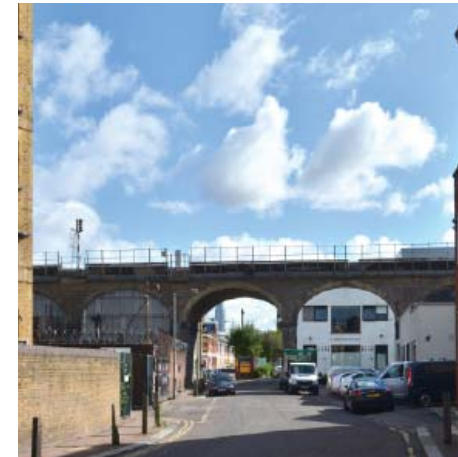
8 - Viaduct and the Site Entrance
