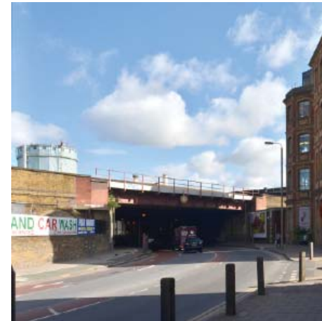
7 - The Viaduct and Gas Station
