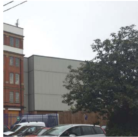
3 - New storage building along entrance
