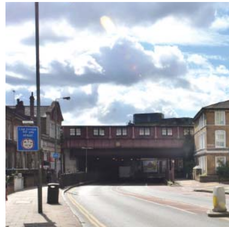
6 - Queenstown Road Station
