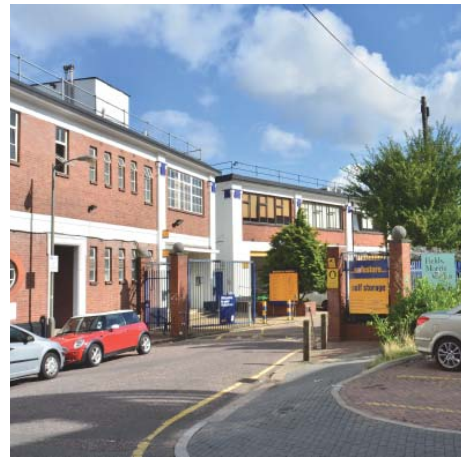
4 - Workshops to the north
