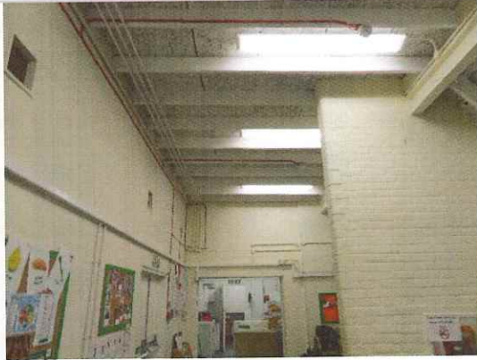
Photograph 1. Underside of roof in the centre
