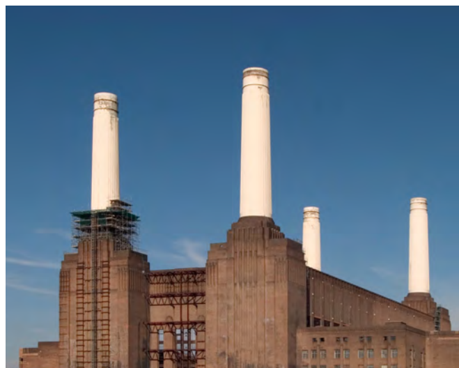
Wandsworth has historically developed around its river frontages, with Battersea Power Station on the River Thames now the centre of one of the largest regeneration projects in Europe
