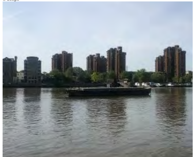
Fig.520: Montevetro Management Building public realm looking north west, Photo
