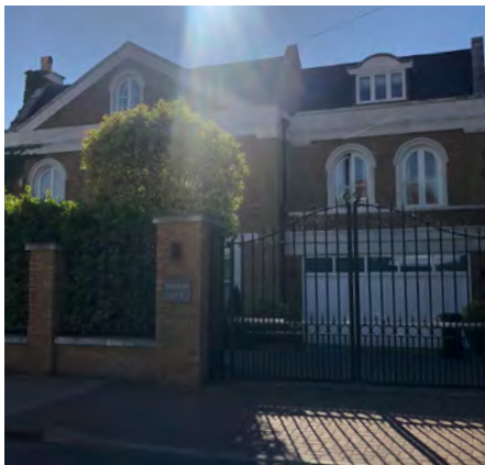
Fig. 161: Large detached house on Roedean Crescent
