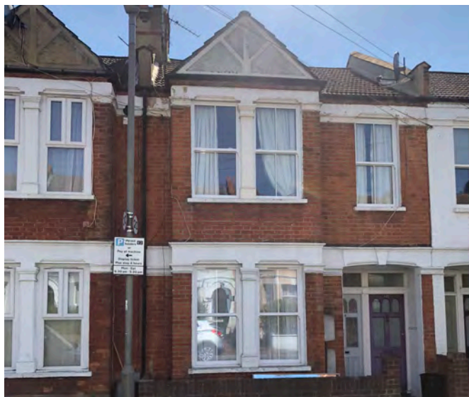
Fig. 179: Two storey period terraces on Totterdown Street
