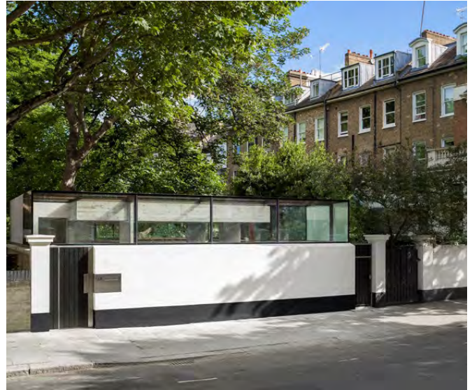
Fig.451: Earl's court house - A contemporary design on a small site that discreetly slots into a conservation area.
