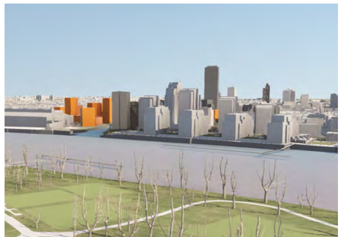
Fig. 406: Oblique view towards the Wandle Delta masterplan from Hurlingham Park. The consented masterplan blocks would provide a visual step down from existing taller riverside development, and protect the river frontage itself from being over-developed
