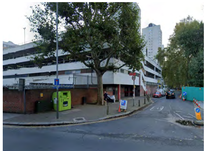
Fig. 374: View into the zone from the junction of Buckhold Road/Neville Gill Close to the north west
