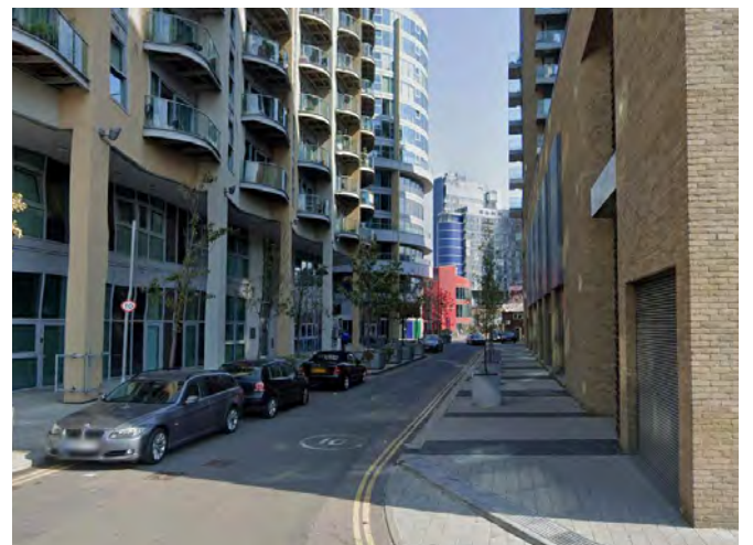
Fig. 273: View north east across the zone from Bridges Court Road
