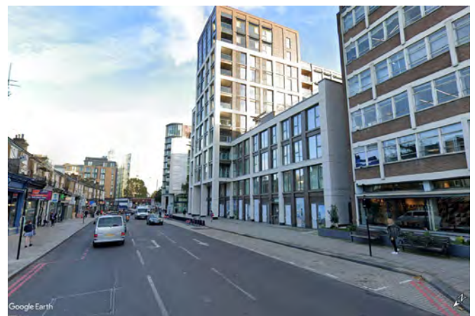
Fig. 345: Buildings up to 12 storeys on Upper Richmond Road near the junction with Carlton Drive
