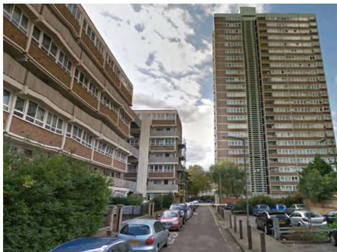
Fig. 256: 24 storey Totteridge House and blocks on Yelverton Road
