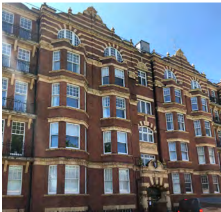
Fig. 129: Kenilworth Court mansion blocks with views across Putney Bridge and the river
