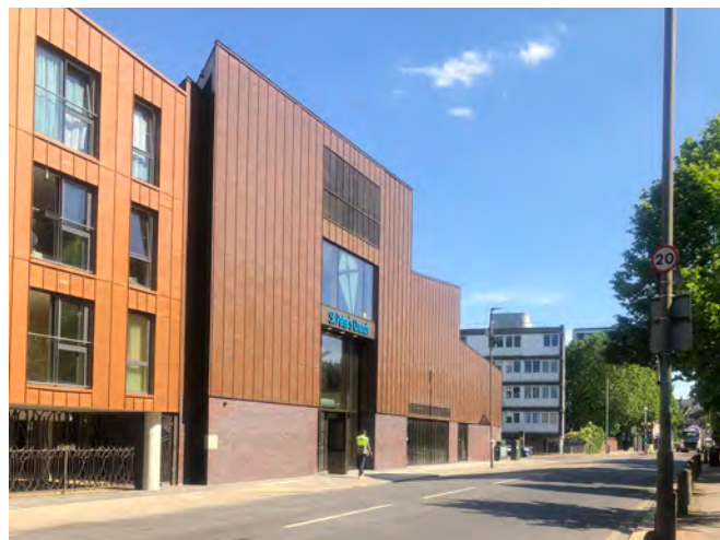
Fig. 247: Buildings including St Peter's Church on Plough road along the western boundary
