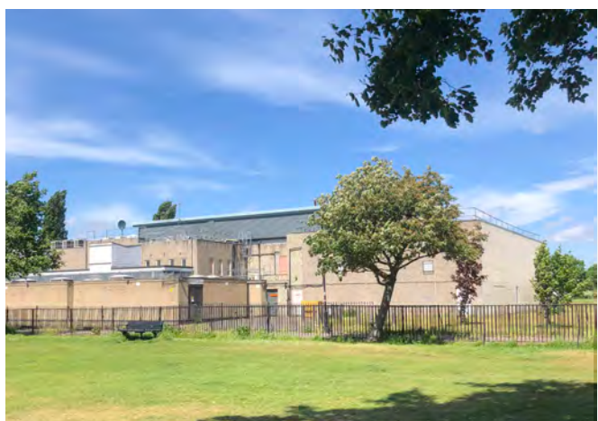
Fig. 502: Large floor plate sub station in Wandle Valley
