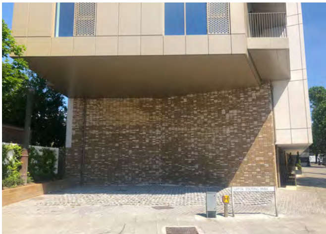
Fig. 420: An example of a poor ground floor frontage at a development on the corner of Balham High Road and Upper Tooting Park
