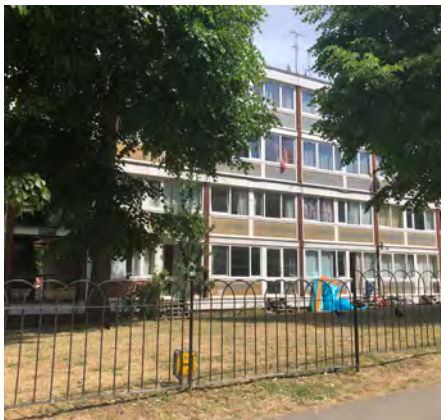
Fig. 167: Bland amenity grass in front of the 4 storey block creates a poor frontage to Danebury Avenue
