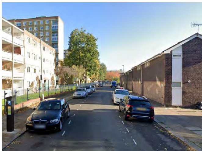
Fig. 263: Existing 4 and 11 storey blocks on Blondel Street
