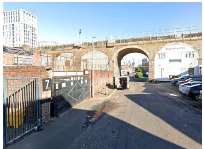
Fig. 296: View east along Ingate Place in the north of the zone
