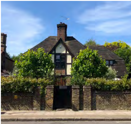
Fig. 141: 1930s Old English cottage style house in Portinscale Rd, East Putney Conservation Area
