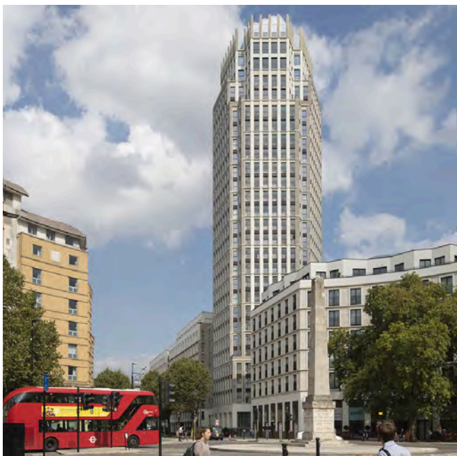
Fig. 412: Blackfriars Circus, 'The use of brick cladding on this tall building gives it a character that fits well into its historic surroundings, and a texture that is human scale and tactile where the building meets the ground.'
