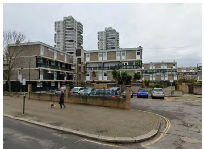
Fig. 267: Existing towers behind car parking area on Westbridge Road
