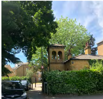
Fig. 147: House on Windlesham Grove provides a historic reminder of the former Victorian lodge
