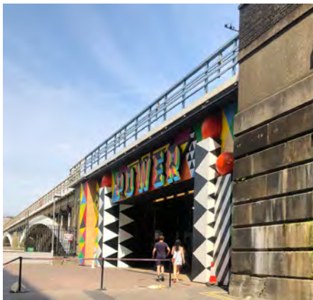
Fig. 77: Colour and vibrancy created by artistic Grosvenor Arch gateway under Battersea Bridge
