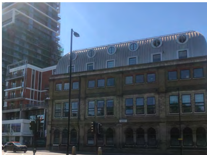
Fig. 272: Locally listed Candlemakers Apartments, York Road
