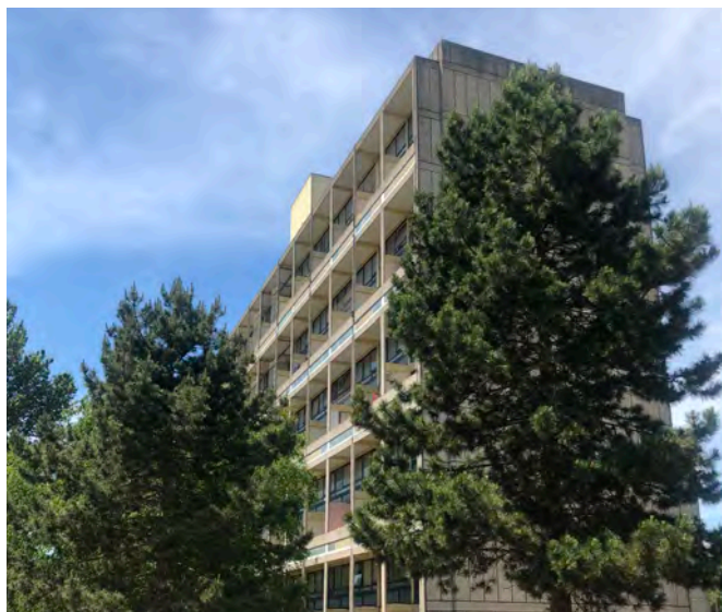
Fig. 165: Grade II* listed Denmead House in Alton Conservation Area, surrounded by Scots Pine trees part of the parkland setting
