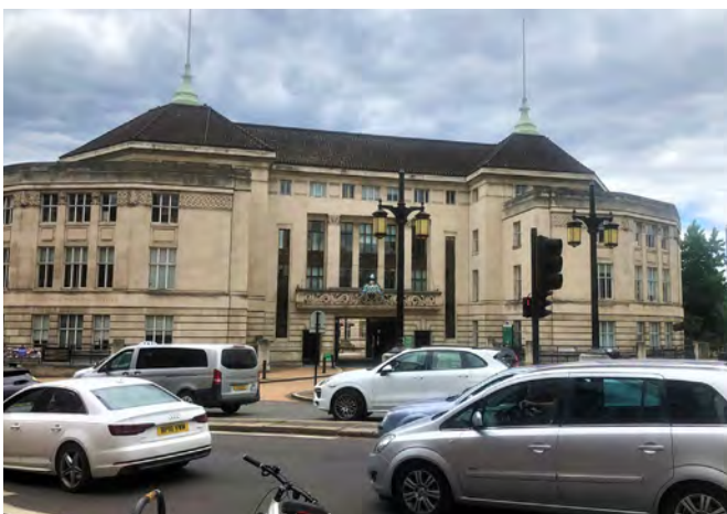
Fig. 506: Wandsworth town hall
