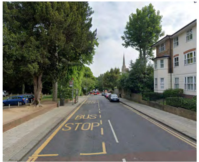
Fig. 643: Alton Road looking north east Photo
