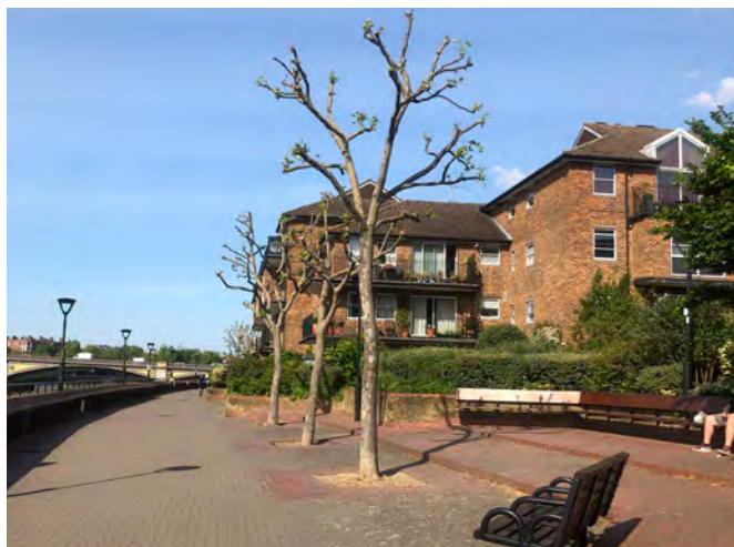
Fig. 279: View along the Thames Path with the tall building zone to the right characterised by 3-4 storey 20 th century development at present
