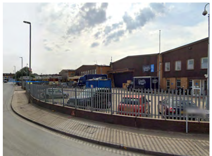
Fig. 325: View east across the site from Riverside Road. Existing industrial buildings are mostly 2 storeys.
