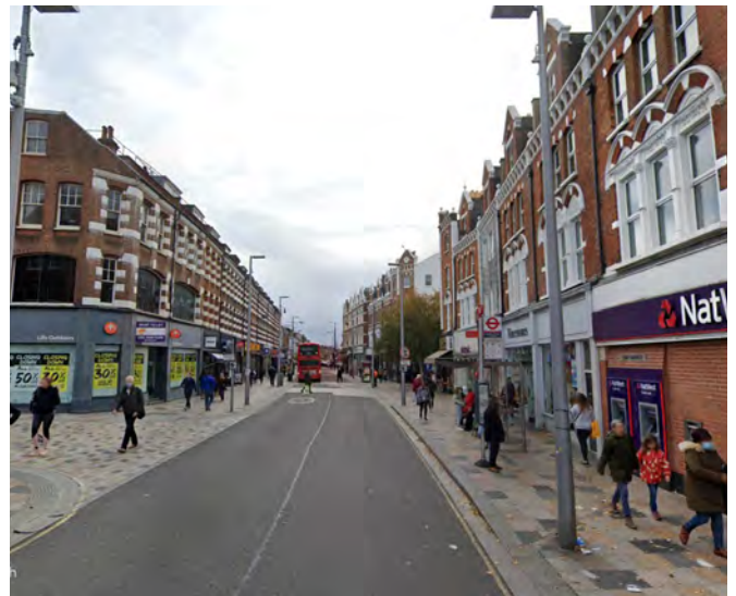
Fig.544: Falcon Rd looking south Photo © Google
