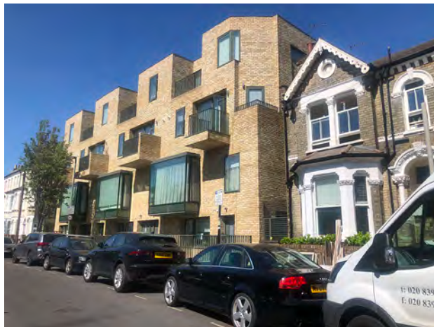
Fig. 475: 4-8 Hafer Road scheme photo
