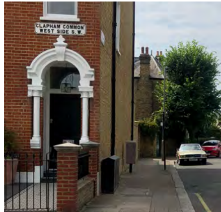
Fig. 96: Interesting white plaster details and quality red brick finishes near Clapham Common
