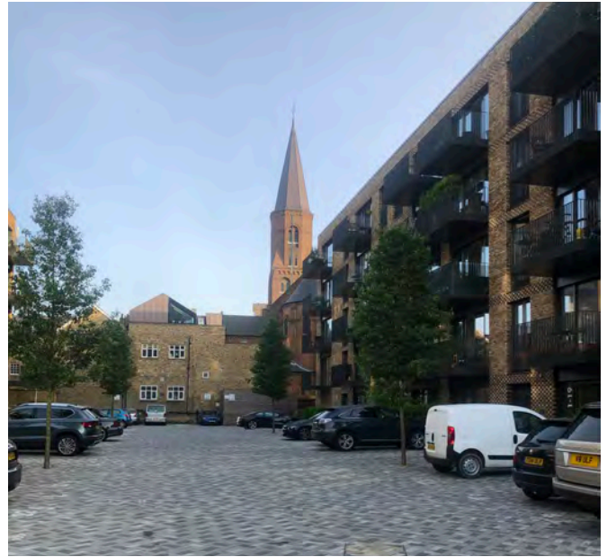
Fig. 414: This new development in Granfield Street successfully responds to the nearby Grade II Church of the Sacred Heart in Battersea Square Conservation Area, through use of high quality bricks, and use of subtly different coloured bands of bricks. Successful use of sensitive architectural detailing and its subservient scale to the church landmark, alongside the courtyard space which frames views to the spire.
