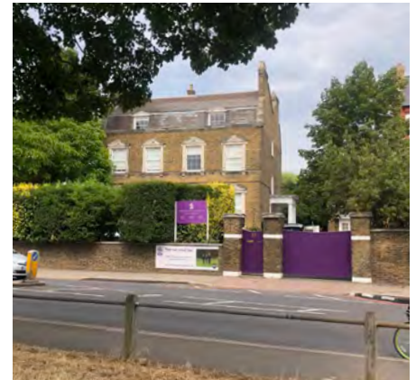
Fig. 97: Springwell House (grade II listed), a Georgian house fronting Clapham Common
