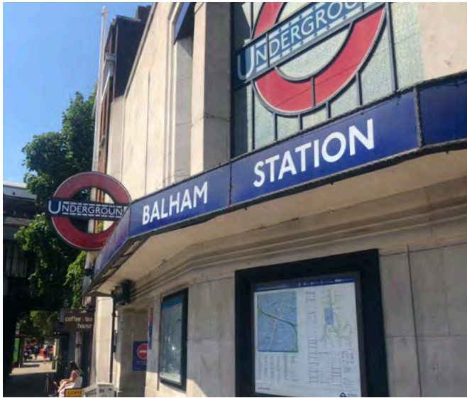
Fig. 49: Balham Station (grade II), designed by Charles Holden and built from Portland stone in 1926. Twin buildings straddle Balham High Road.
