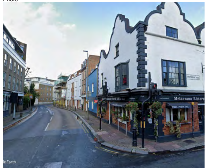
Fig.521: Battersea Church Rd looking north, Photo © Google
