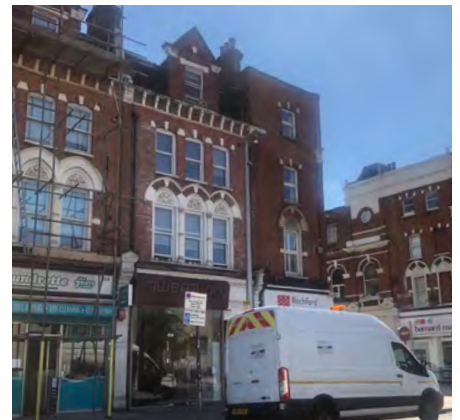
Fig. 91: Typical 4 storey red brick shop terrace on Lavender Hill
