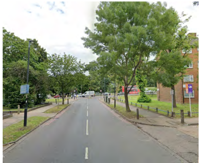
Fig. 659: Aldrington Road looking north Photo
