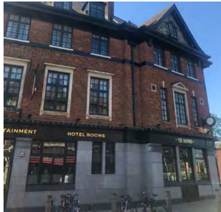
Fig. 52: The Bedford pub is a strong landmark on the corner of Bedford Hill/Balham Station Road
