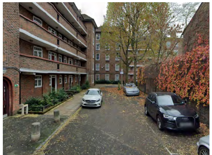
Fig. 289: 5 storey blocks on Savona Street
