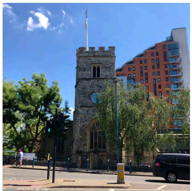
Fig. 415: St Mary's Church next to Putney Bridge is overwhelmed by the adjacent Putney Wharf Tower
