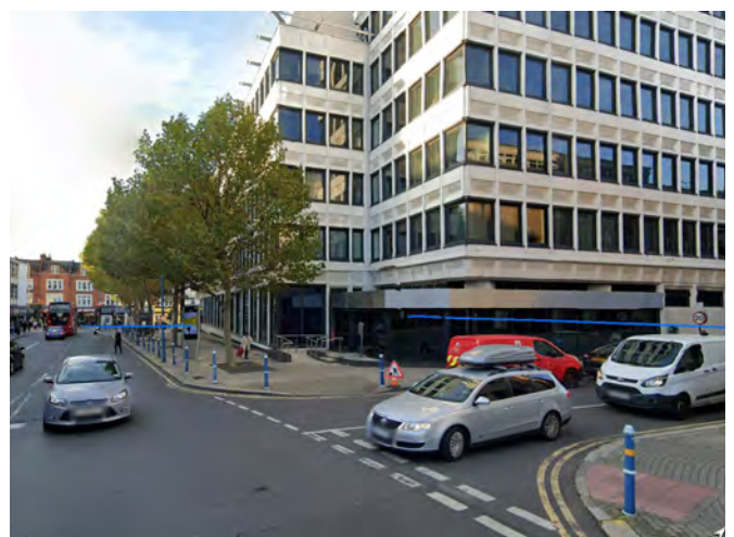
Fig. 334: View into the zone from Putney Bridge Road
