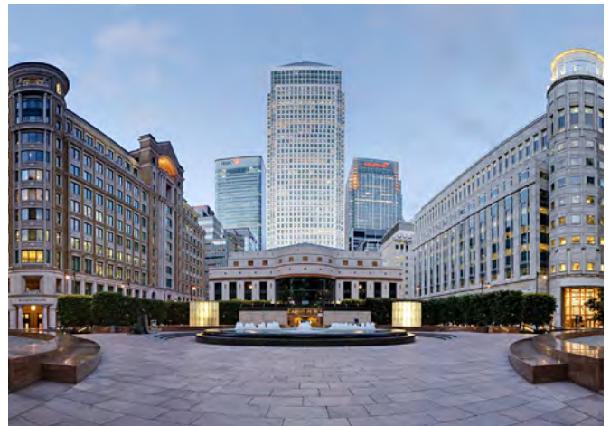
Fig.407: One Canada Square, Canary Wharf was designed as a landmark with views framed by surrounding background buildings © Photo by DAVID ILIFF. License: CC BY-SA 3.0
