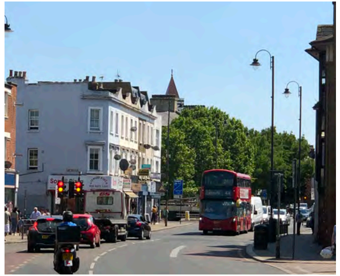
Fig. 649: Mitcham Road facing south east Photo
