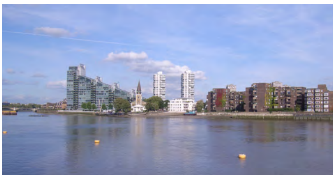
Battersea's mixed riverside frontage
