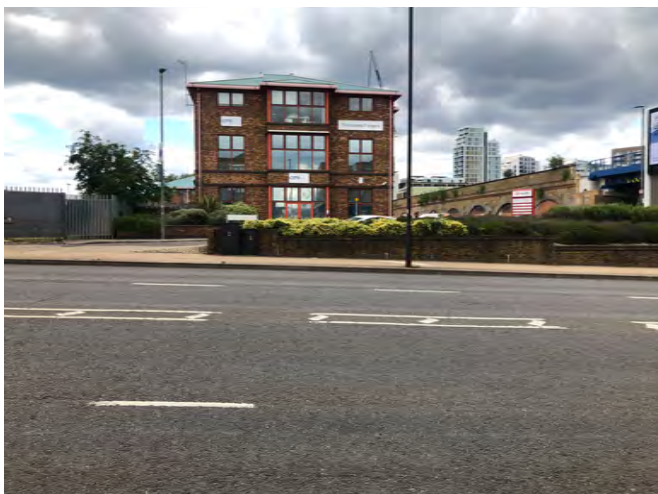
Fig. 388: Office building in the north east of the zone, from Swandon Way
