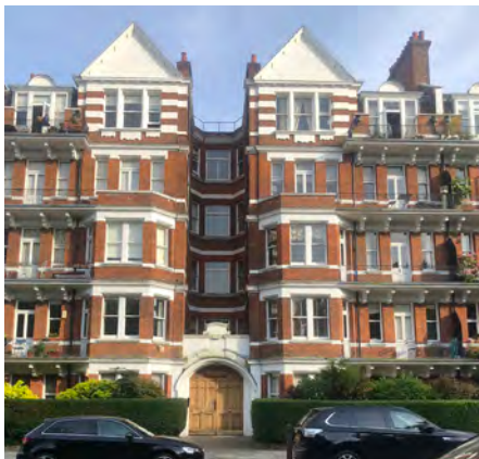
Fig. 83: The 5 storey Prince of Wales Mansions (locally listed) provide a robust frontage to the park
