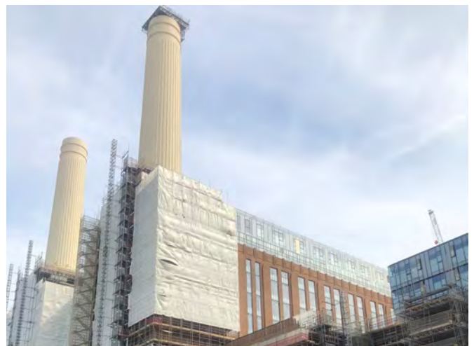
Fig. 286: Battersea Power Station undergoing redevelopment
