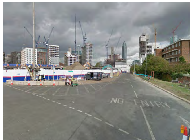
Fig. 303: View north along the southern boundary of the zone, with 5 storey blocks in LB Lambeth to the right of the view and towers in Vauxhall ahead
