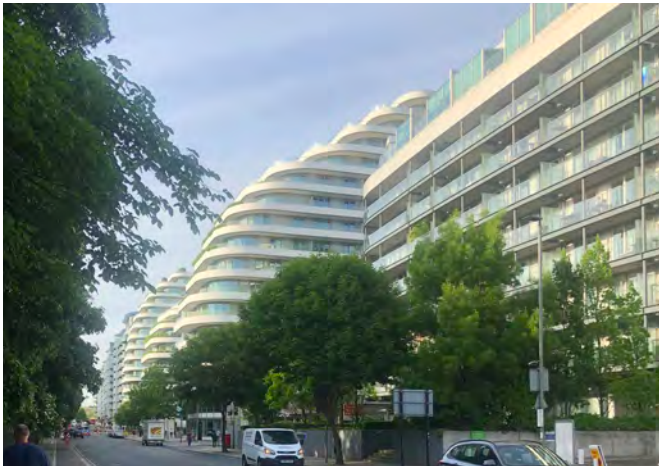
Fig. 495: High-rise flats in Nine Elms
