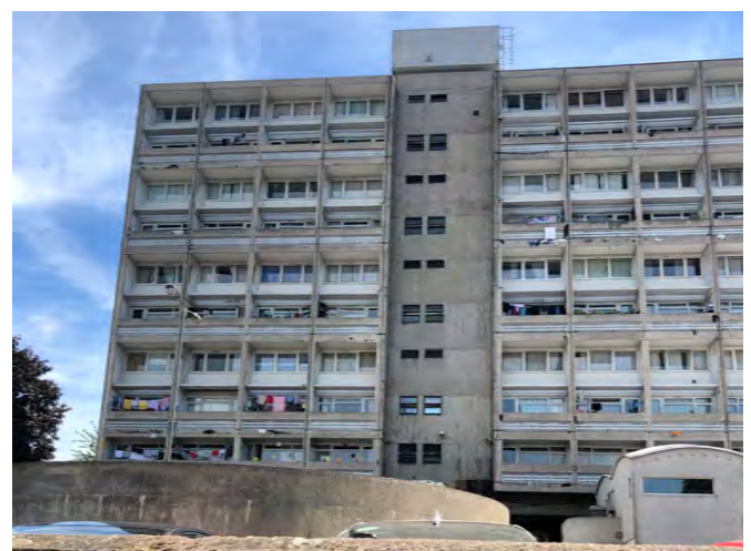
Fig. 349: Roehampton library on Danebury Avenue
