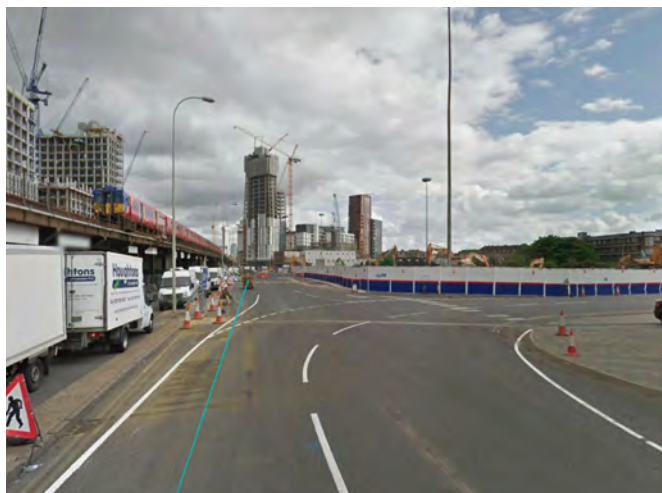
Fig. 302: Looking along the northern boundary of the zone beyond the hoarding to the right of the view, and towards towers in Vauxhall
