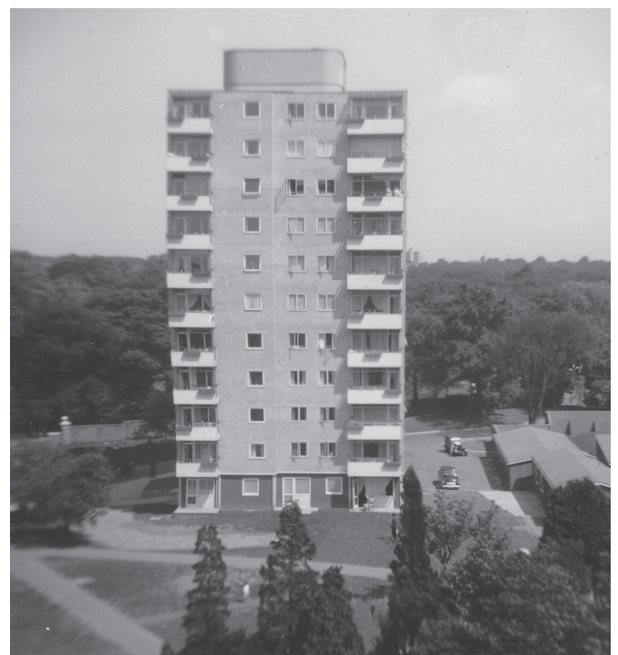
Fig.20: Alton East Estate, 1957 © Wandsworth Heritage Service
