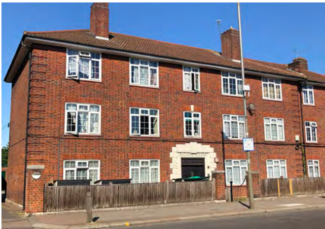
Fig. 490: Low-rise flats house in Tooting
