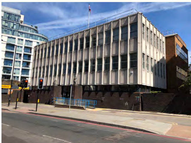
Fig. 344: Between the railway line and Woodlands Way
