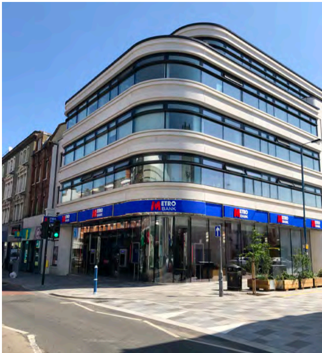
Fig. 456: Art Deco style new build along Putney High Street, with the frontage expressing itself to mark a strategic junction
