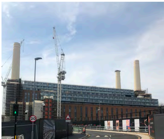
Fig. 75: Battersea Power Station during redevelopment
