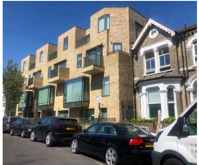
Fig. 453: New terraced homes adjacent to period terraces at Hafer Road
