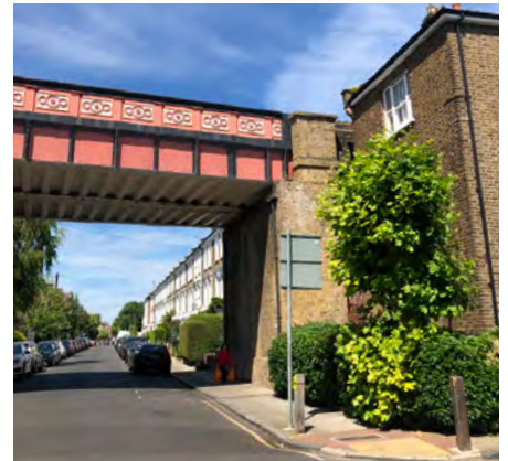
Fig. 143: Railway bridge at Fawe Park Road
