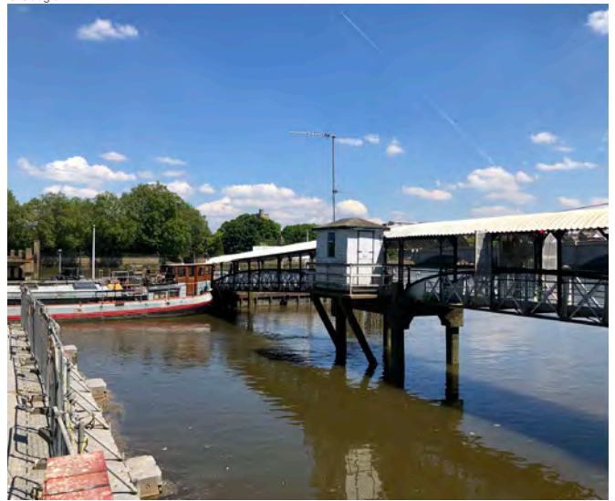
Fig.588: Putney Emankment looking north Photo
