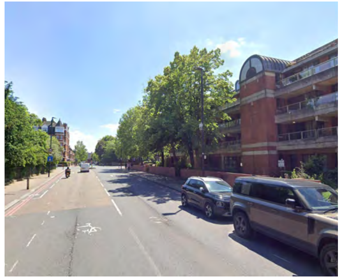
Fig. 534: Albert Bridge Rd looking south, Photo © Google
