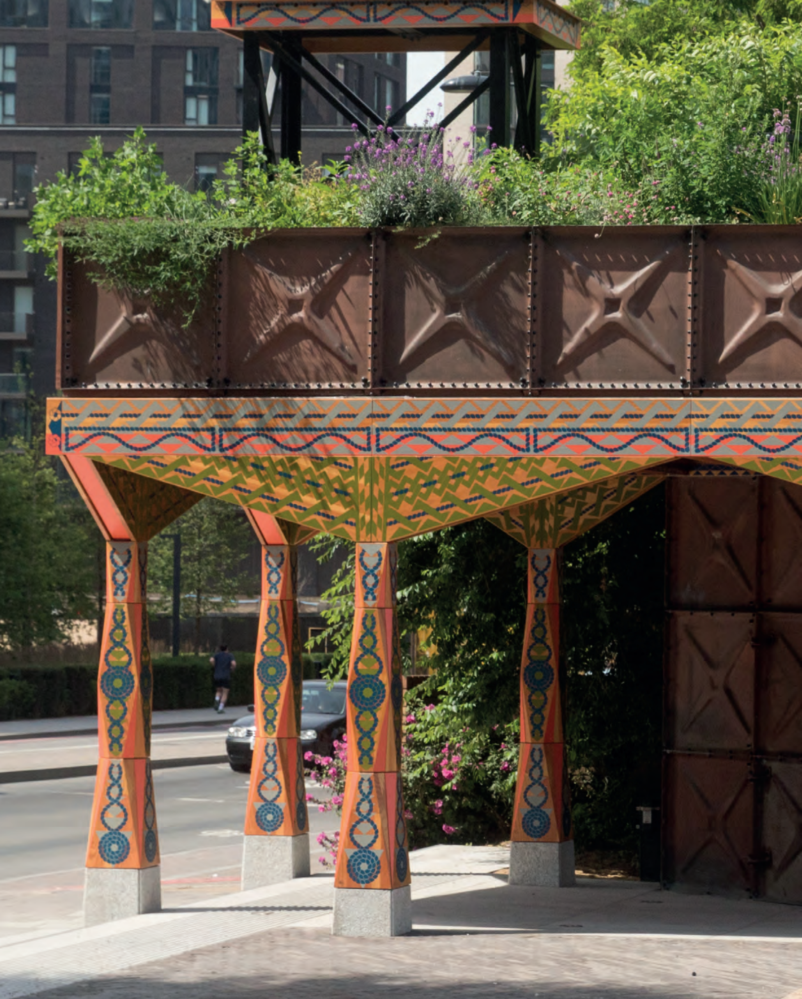
The Nine Elms Pavilion, designed by Studio Weave and artist Linda Florence, opened in June 2018. It has created a new public space along the river supporting events and performances to take place, as well as giving residents and visitors a place to relax by the river. The raised garden provides an additional patch of greenery offering a haven to insects.
